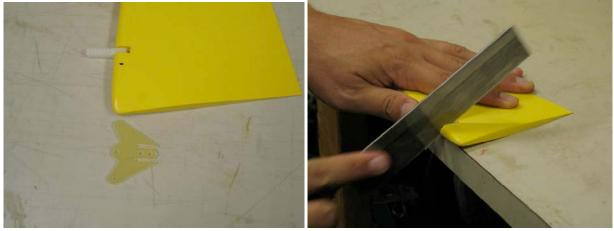
19. When satisfied with the fit of the control horn (make sure both holes in the control horn are equidistant from the center of the hinge), glue it into the rudder using thin CA or epoxy.
